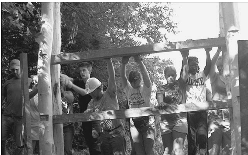
Student volunteers support the new structure while Bob McNamara and Nick Gavrielides ensure that uprights are plumb.
