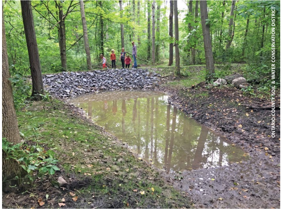
The Land Trust supported a joint project between the Ontario County Soil & Water Conservation District and the Town of Geneva to install retention ponds at the Kashong Conservation Area in Geneva. The ponds are designed to control flooding and erosion caused by stormwater runoff at this conserved area where the Land Trust holds a conservation easement.
