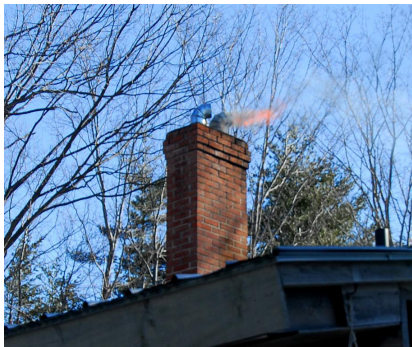
Chimney fire resulting from creosote build-up
