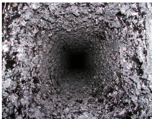
Creosote lining an interior chimney wall
