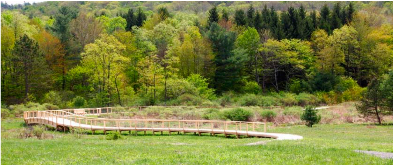
The new boardwalk at the Roy H. Park Preserve/Tom Reimers
