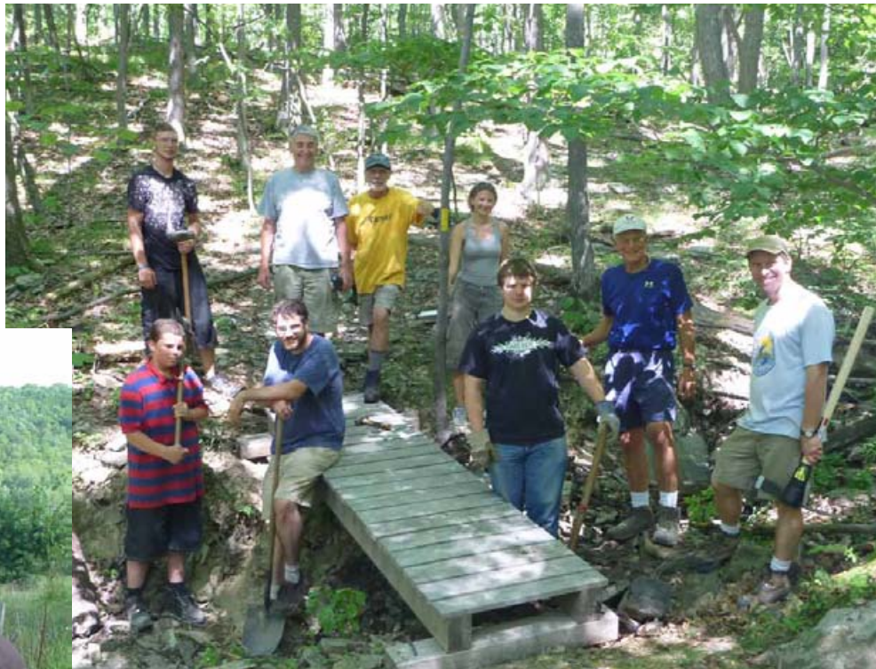
Replacing a bridge at the Steege Hill Preserve
