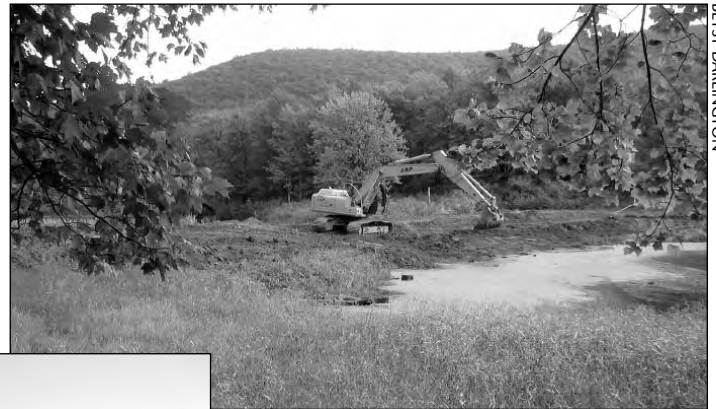
The new Coleman Lake dam, with its gentler slope, will be lower and broader and provide the lake with a wider wetland edge, attracting a greater variety of fauna from around the area.
