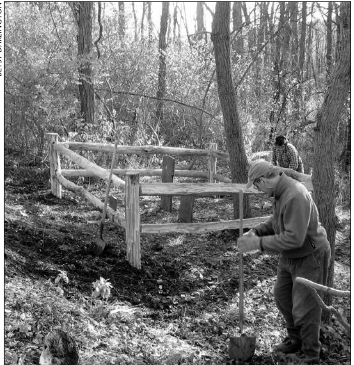
Member and volunteer Bill Hecht (foreground) with Stewardship Ecologist Mark Whitmore at the Salmon Creek Bird Sanctuary, completing work on the new fence that surrounds the graves of two Revolutionary War veterans. Post holes for the fence were dug by Cornell fraternity members of Psi Upsilon.
