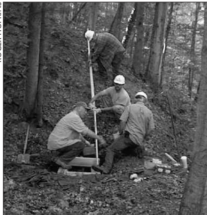
Land Trust volunteers work with volunteers from Dominion Transmission to install steps at the new Kingsbury Woods Conservation Area.
